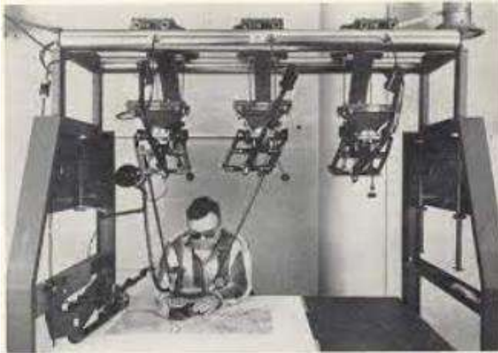
Fig: Man plotting map using stereoplottter
